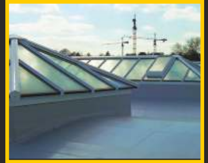
Suitable for Commercial Roofs
